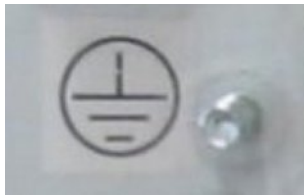
Fig. 19: Grounding stud marked with PE symbol
